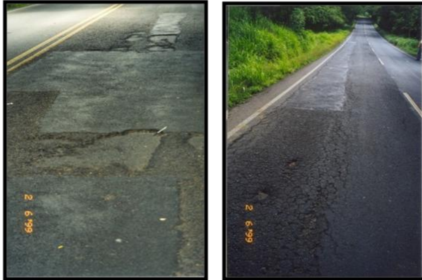
Figure 2. Condition of the highway system in 1999
