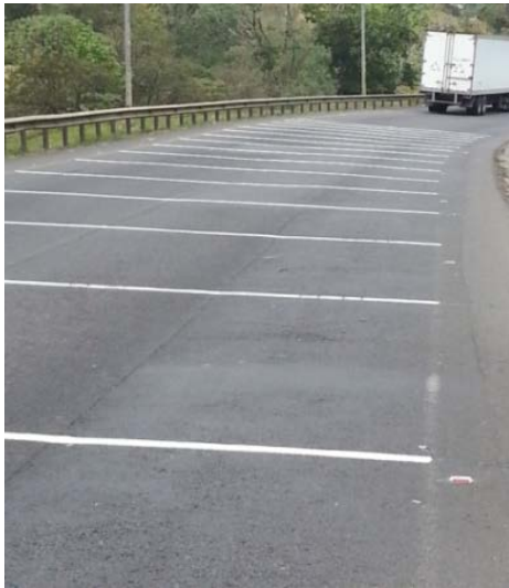
Figure 5 – Installation of markings at Sites 2.
