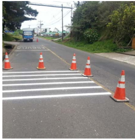
Figure 6 – Installation of markings at Sites 3.
