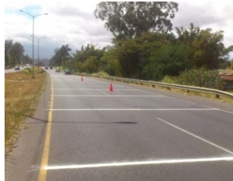
Figure 3 – Installation of markings at Site 1.
