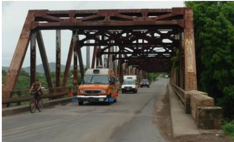
(a) Safety condition on bridges
