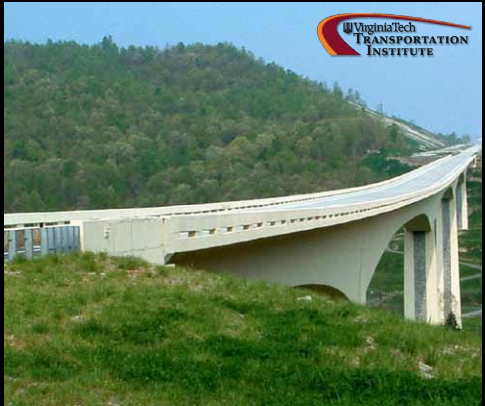
Fig. 1. Smart Road Bridge
