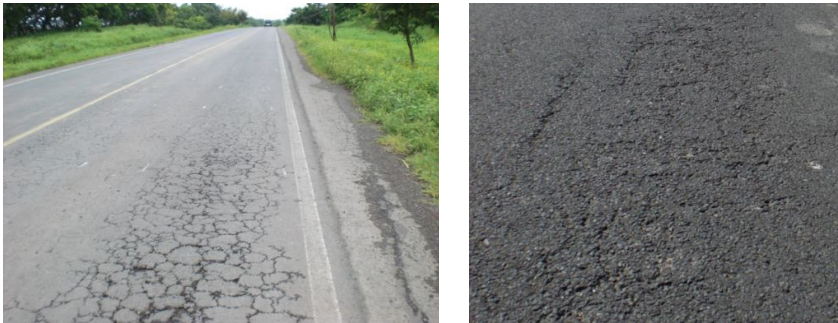
Figure 17. Route conditions before the intervention.
