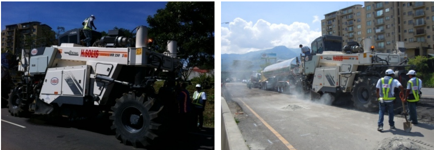
Figure 15. Equipment used in stabilization process in Route 39 in Costa Rica.
