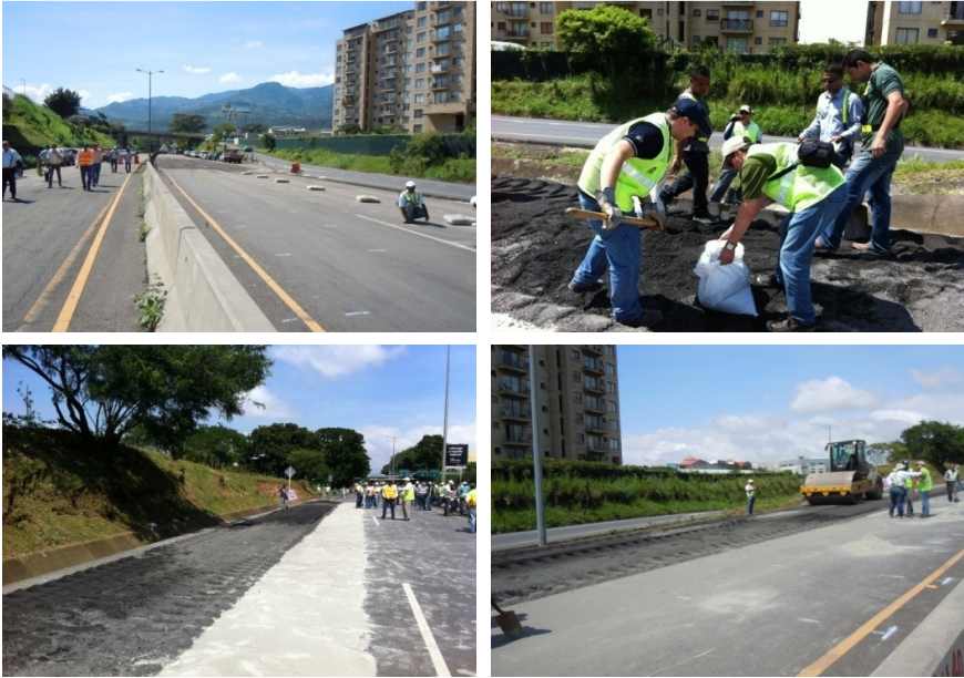
Figure 14. Stabilized section with foamed asphalt in National Route 39 in Costa Rica.
