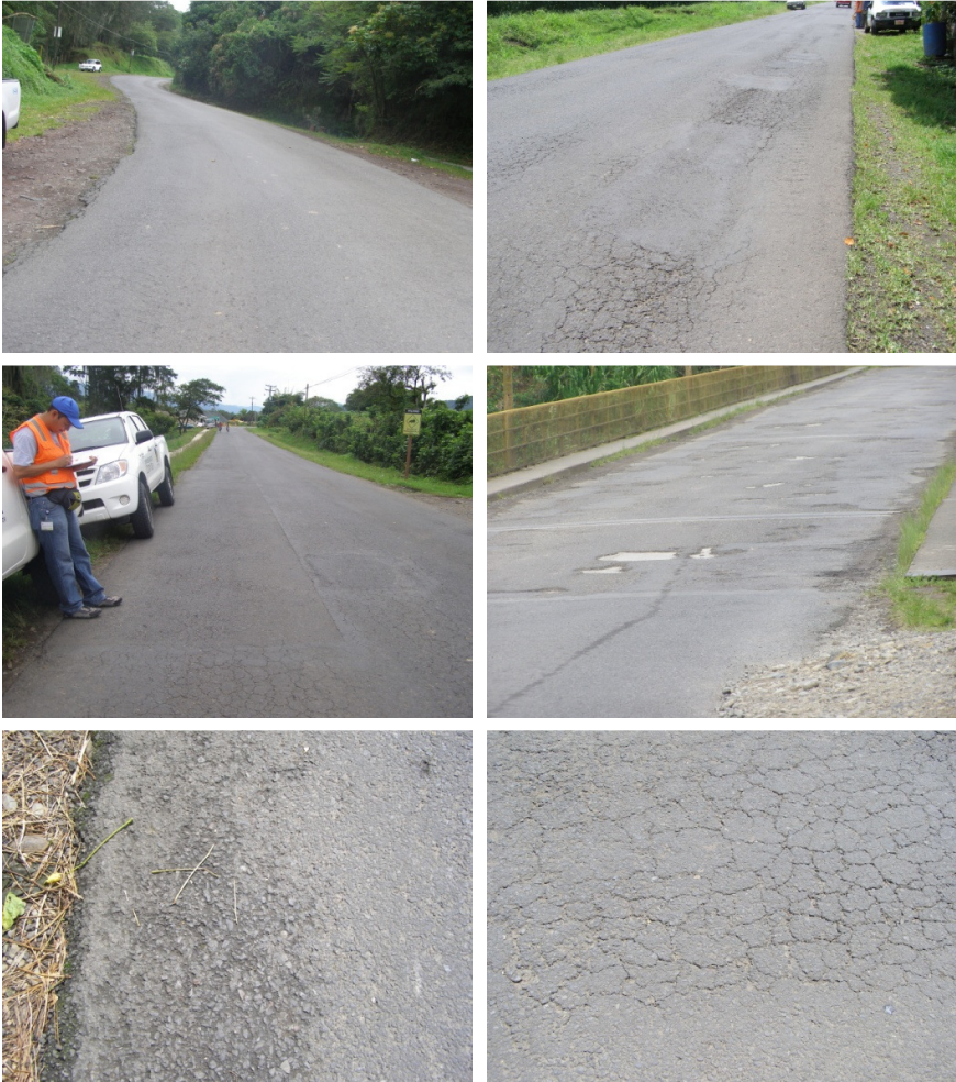
Figure 13. Stabilized section with foamed asphalt in National Route 244 in Costa Rica.
