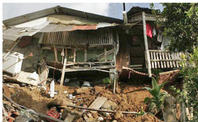
Figure 2. House affected by Cobano earthquake in 1990
