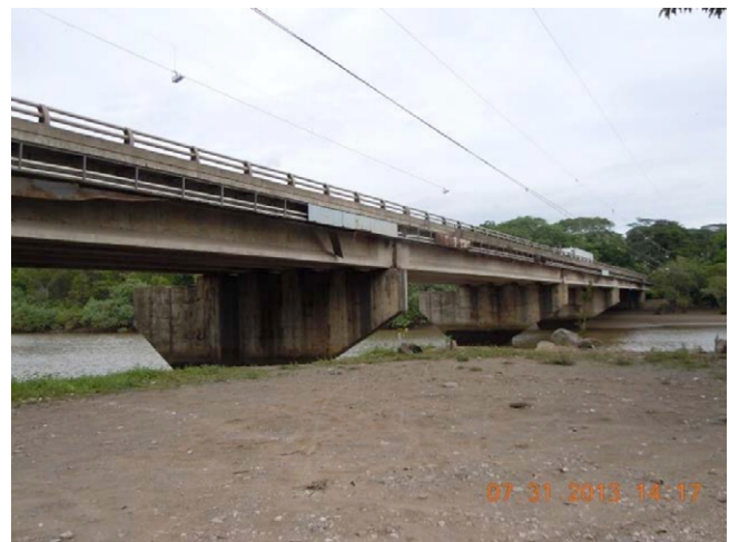
Figure 4. Longitudinal and lateral view of the Barranca bridge
