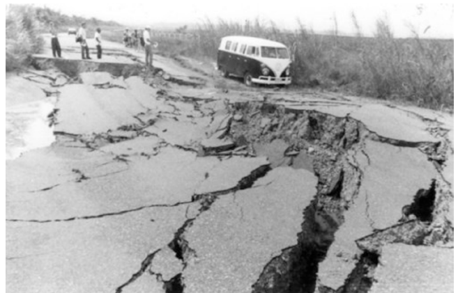
Liquefaction occurred by the natural disaster in 1991
