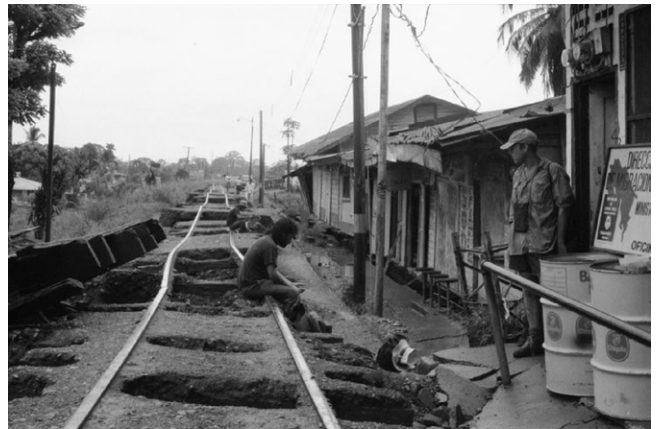
Damage caused by de Limon earthquake
