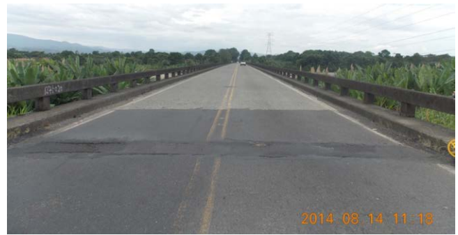
Longitudinal view of the Chirripó River Bridge.
