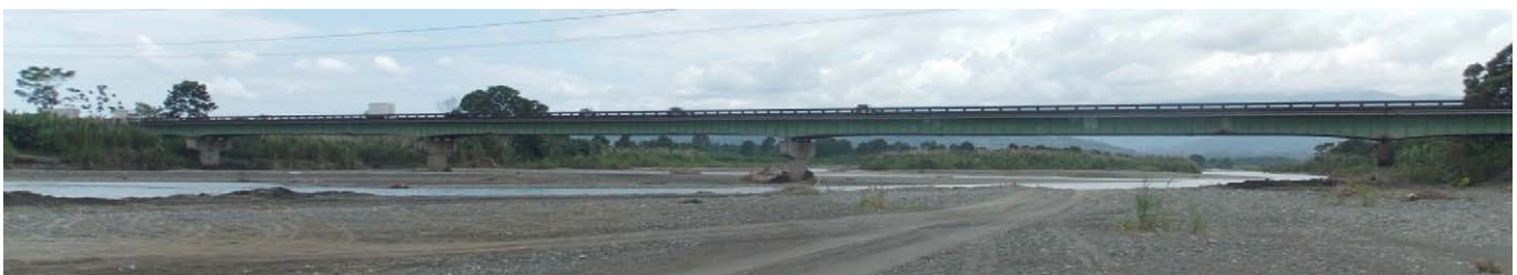
Lateral view of the Chirripó River Bridge.
