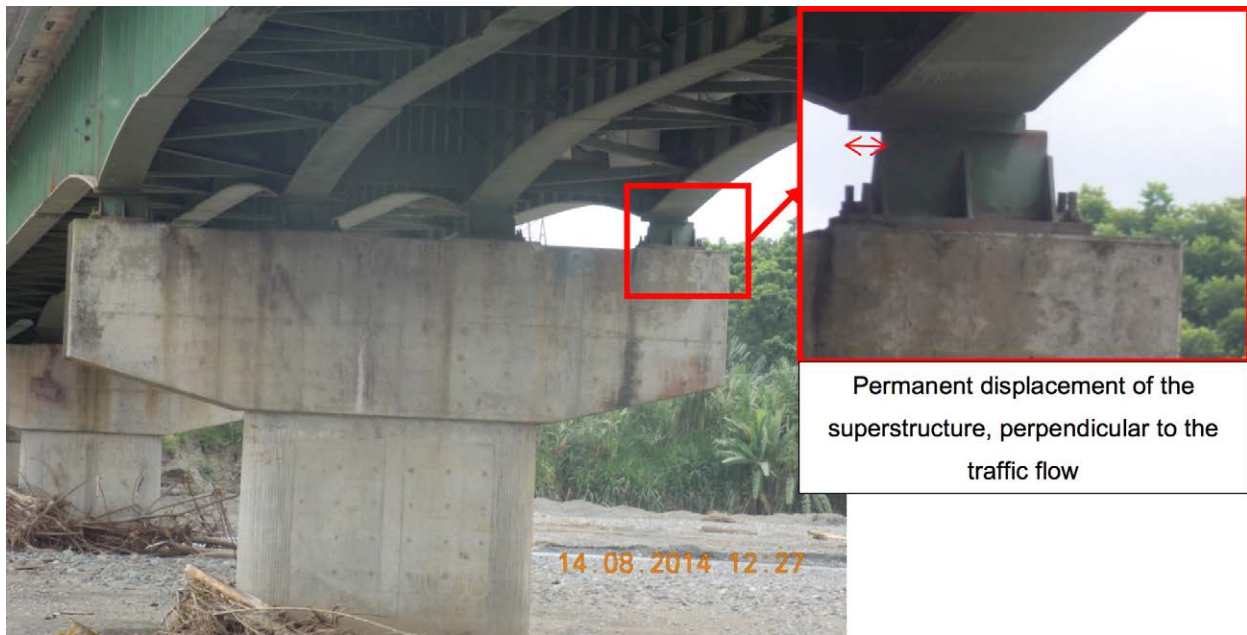
View of the Pier 3 from the east side.
